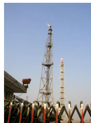
Waste gas recovery system with torch gas in background
