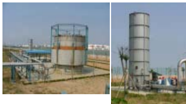
Ground flare, part of a 500kT/y PTA plant
